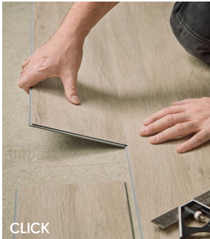
3. No need for adhesive, click and lock the planks into place.
