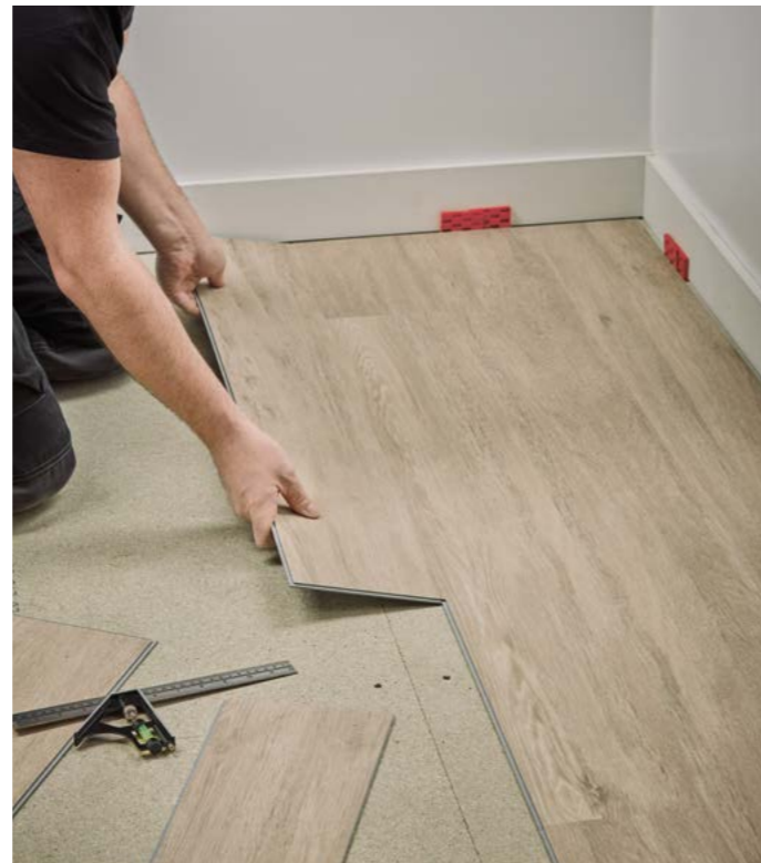
4. Continue to fit the rest of the floor, leaving a 5mm expansion gap. Skirting and colour matched scotias are available, see page 36 for more details.
