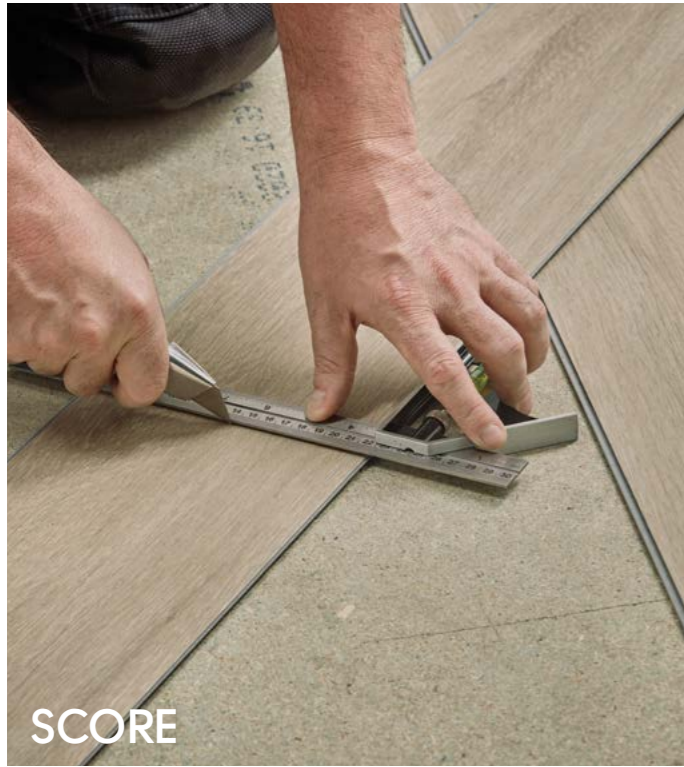
1. Using a knife and a straight edge, score the plank surface.
