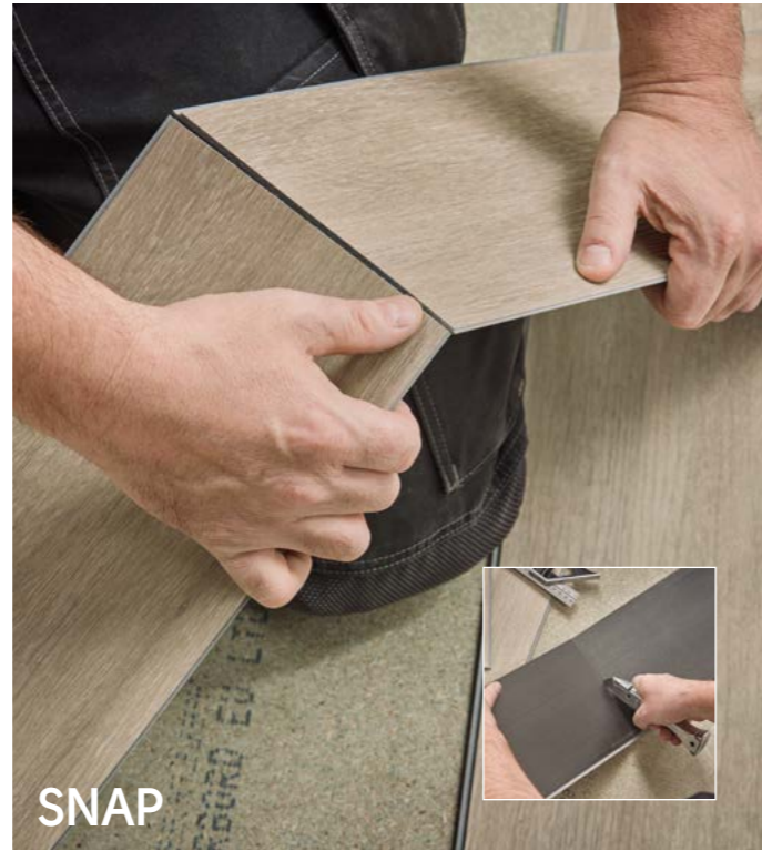
2. Snap the plank and use a utility knife to fully separate.
